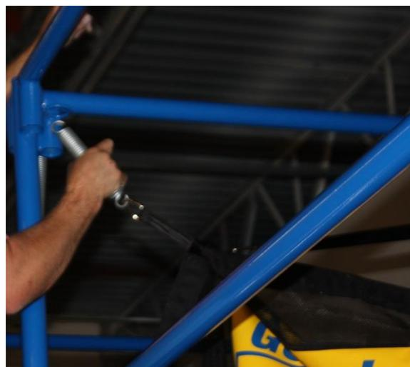
Use the spring tool to stretch the springs if needed. Start with from top and move down. Repeat for the other 3 housings. Ensure that #63L and #63R are on opposing corners.
