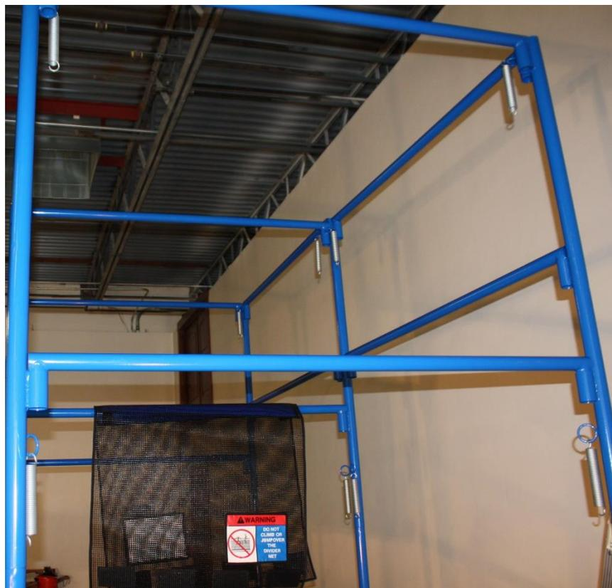
**Step 20:** Prepare the left and right housings – parts #63L (left) and #63R (right) – and find the upper loops for each. Begin by attaching the springs to the top of the structure.
